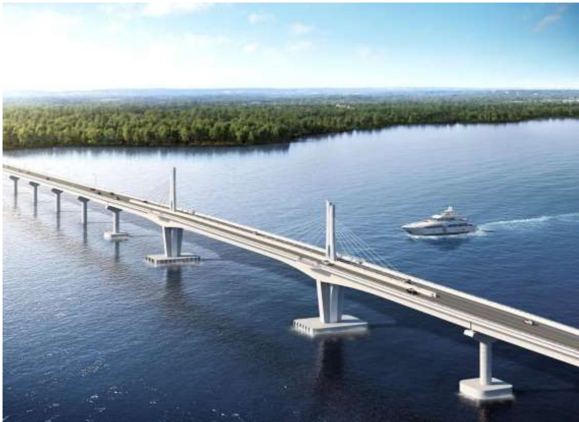
Figure 2. PERSPECTIVE VIEW OF THE PANGUIL BAY BRIDGE
